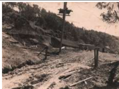
Excavating for new Club House
