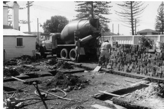
Fig. 42: Construction of footings 1966. Timber verandah enclosure at rear of Store building visible at left. (Source: 2018 CMP, fig. 20. Port Macquarie Museum)
