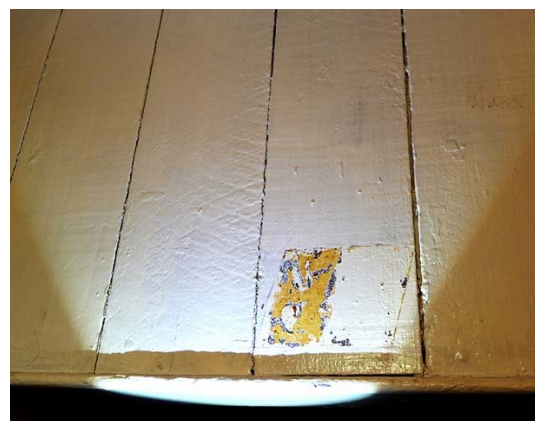
Fig. 22: Some lining boards above the Nursery door appear machine-sawn, and others appear pit-sawn. (Source: Design 5, 2025).
