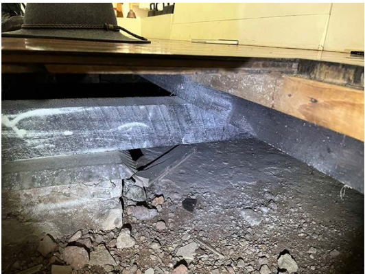
Fig. 13: Compacted earth floor visible in present subfloor space. Looking south from access hatch in Foundation room. (Source: Design 5, 2024).
