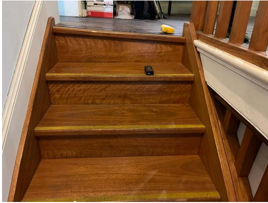
Fig. 64: Existing stair rising up to first floor Parlour, noting deflection in floor level. (Source: Design 5, 2024).
