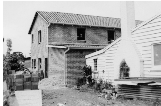
Fig. 43: View of first stage of museum additions nearing completion c1967, looking south. Brick chimney of rear annexe visible at right. Enclosed verandah (centre of view) was demolished as part of the works, and weatherboard annexe enclosure was replaced with brick. (Source: 2018 CMP, fig. 22. Port Macquarie Museum)
