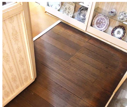
Fig. 21: Evidence of former stair location in first floor. (Source: Design 5, 2024).
