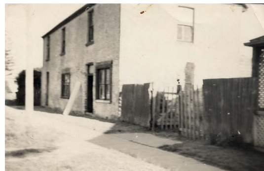
Fig. 37: 1958 photograph. The ground floor door/window on western elevation was already infilled at this time. (Dark mark is the shadow of the
